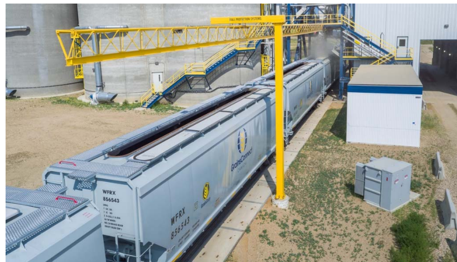
Several new 5,431 cubic-foot hopper cars are spotted for loading at the GrainsConnect Canada facility in Maymont, Saskatchewan. Privately supplied hopper cars, such as those depicted here, have become an important element in the operation of the GHTS today. (Image courtesy of GrainsConnect Canada)
